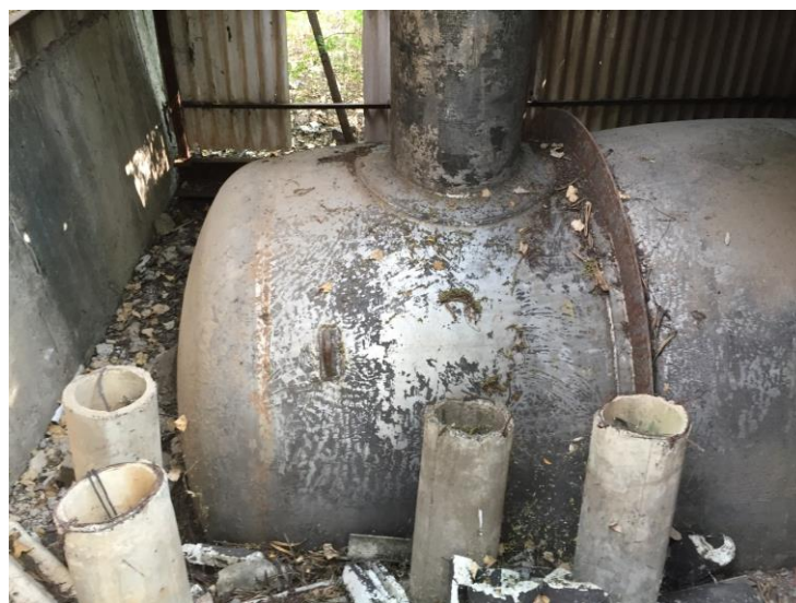
Another view of Tank E641
